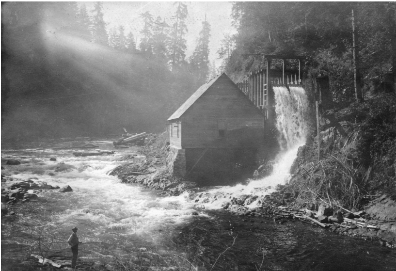
The Kalama River power plant and lower end of the flume, circa 1910. CCHM 1966.0080.0023.
